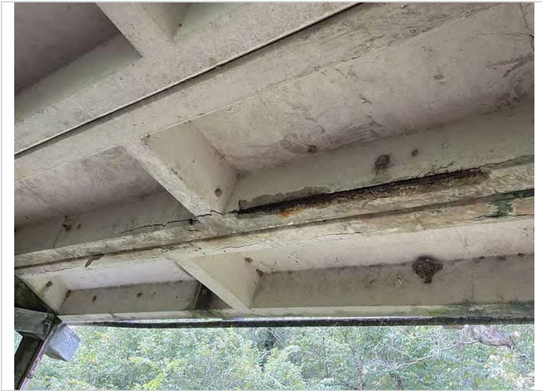
Span #2 PCCS "F" spall to steel
