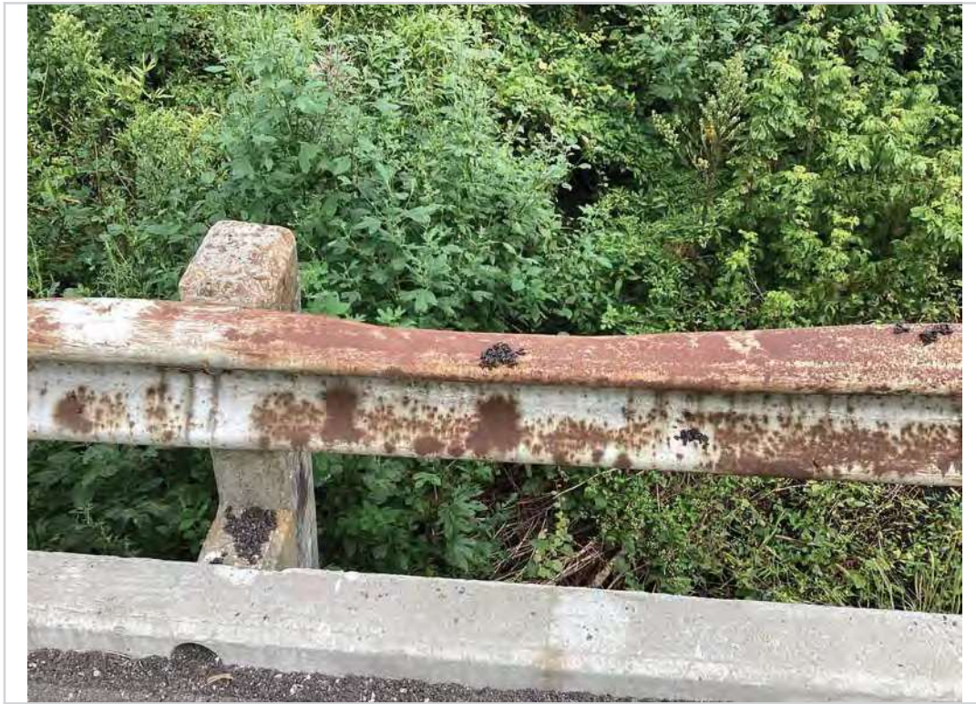
Span 3 rail damage
