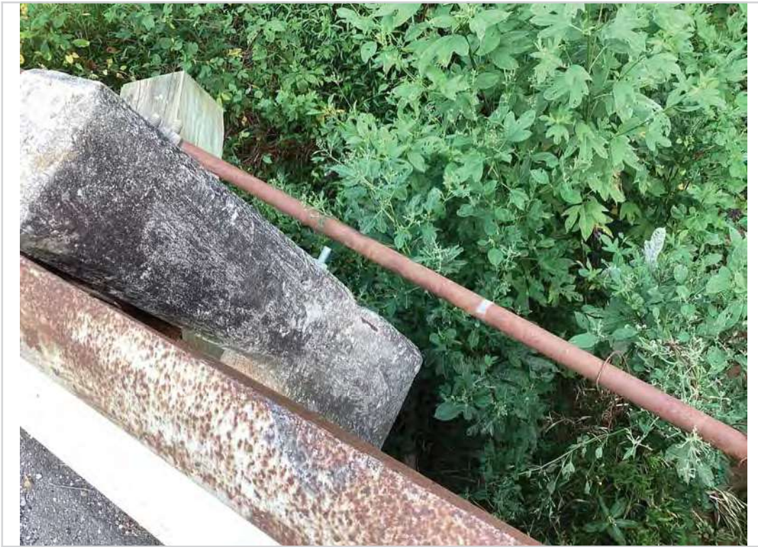
Span 2 post spall to steel
