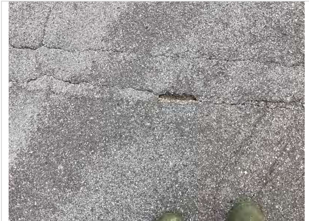
Span 2 spall
