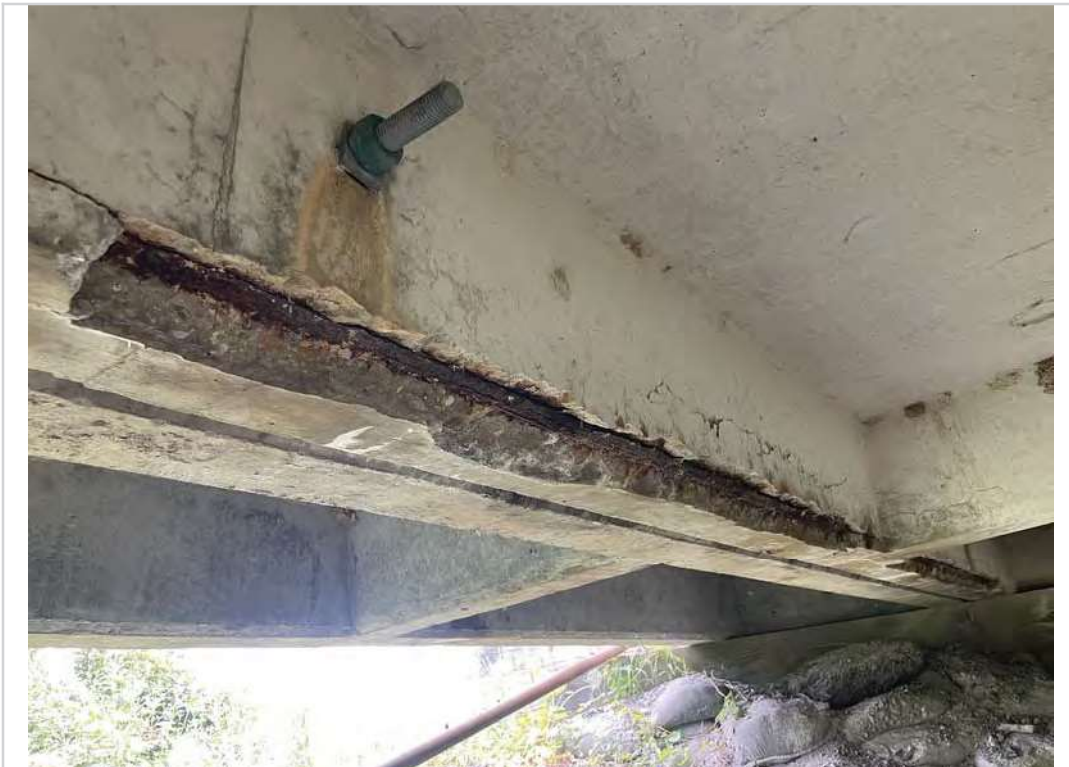
Span #3 PCCS "B" spall to steel
