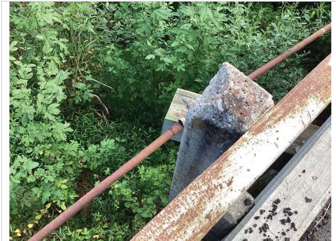
Span 1 post spall
