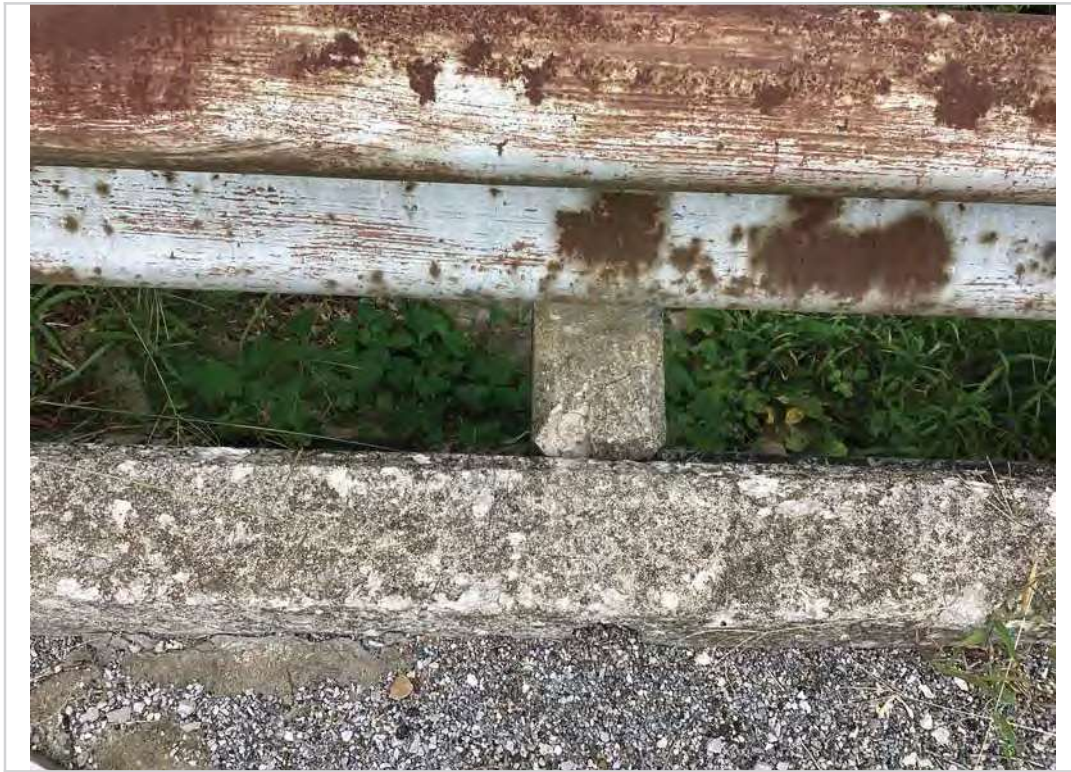
Span 3 post impending spall
