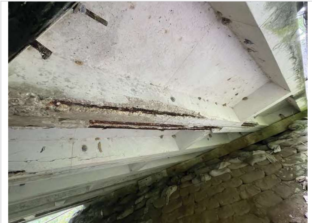
Span #3 PCCS "G" spall to steel
