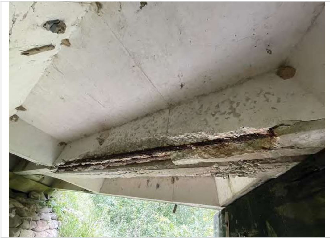
Span #3 PCCS "F" spall to steel
