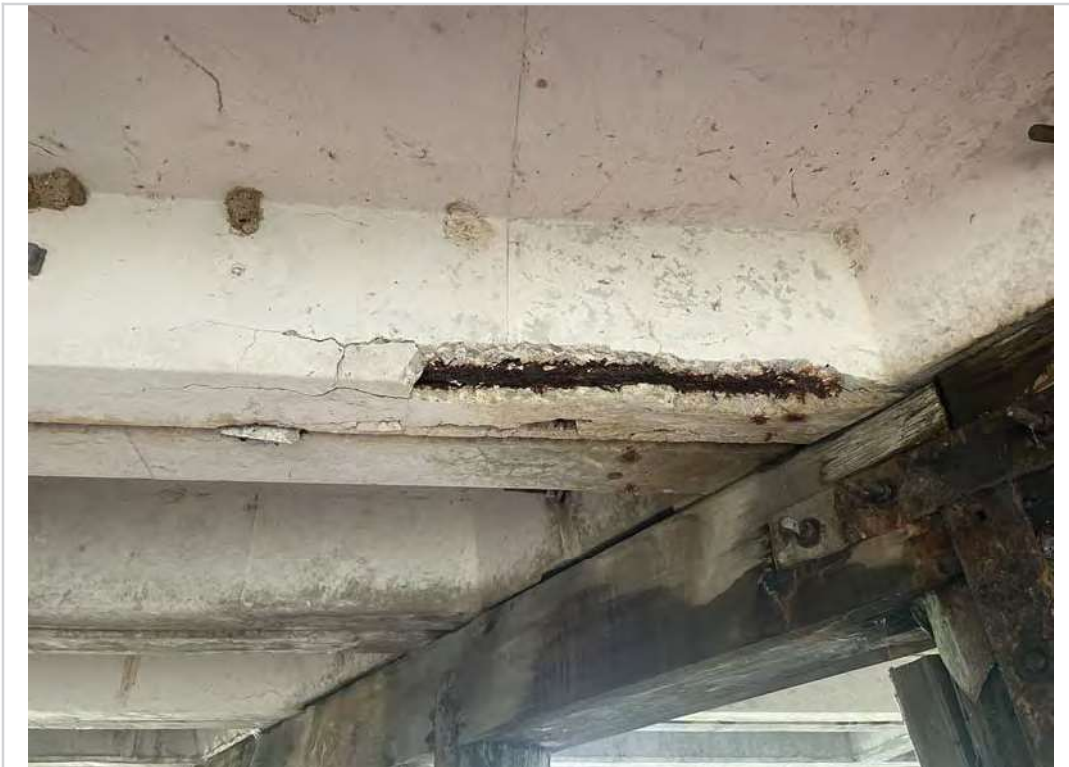
Span #1 PCCS "E" spall to steel
