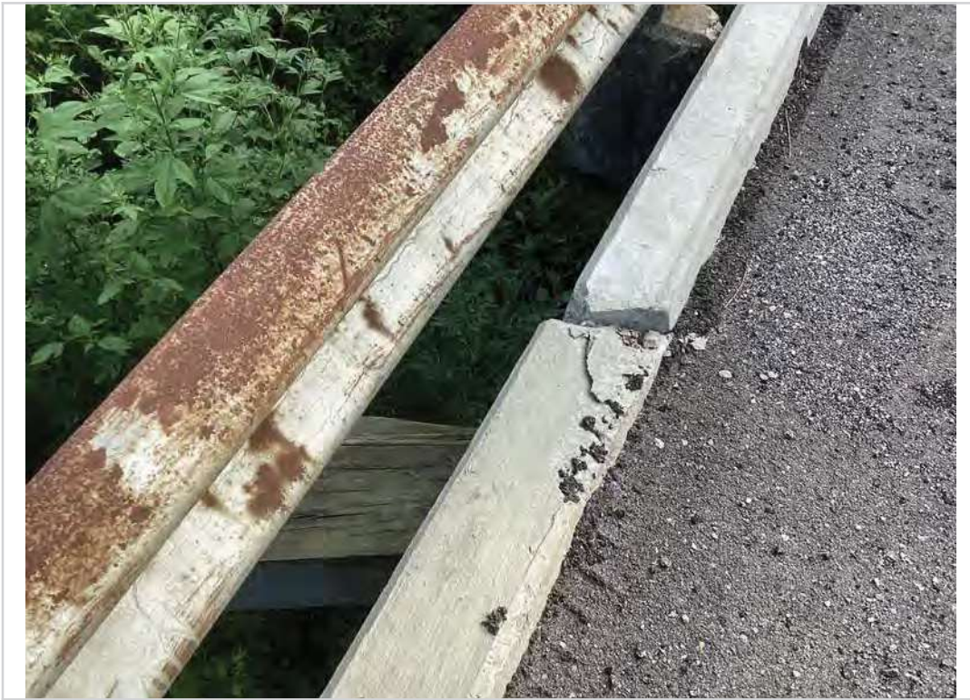
Span 1 curb spall
