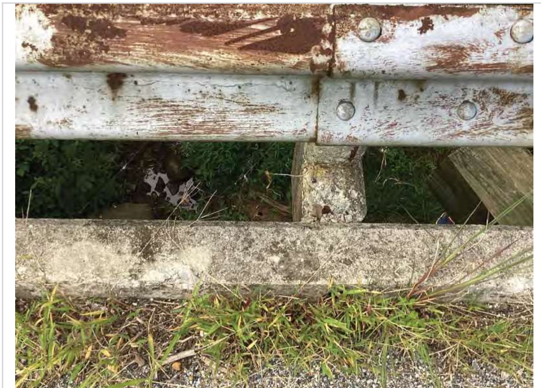
Span 2 post spall to steel
